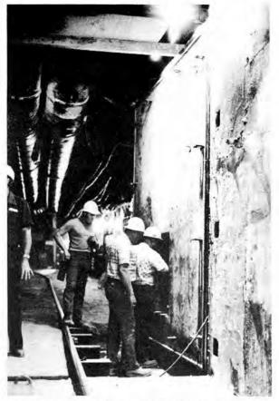
Dick Dye (9131), Hank Kerr (9134), and Hyder Durress (9131) are eyeballing what is called a big door. (not just the opening — the whole thing). It helps seal tunnel.
